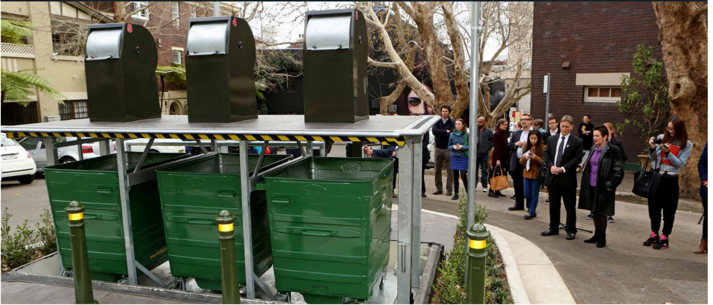
Hydraulic-underground bins in Darlinghurst, Sydney / Image: Damian Shaw
